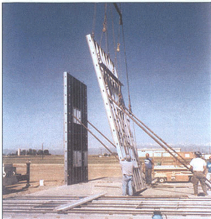
Above and right illustrate the erection process of the MetalStudCrete panels. Below is a view of the completed project which utilized approximately 10,000 sq. ft. of MetalStudCrete panels. Each one was 15' x 24'.
