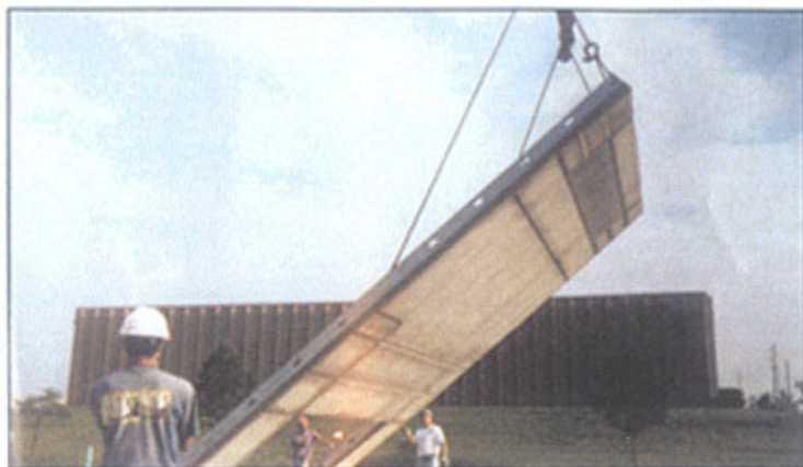
Above and right illustrate the erection process of the MetalStudCrete panels. Below is a view of the completed project which utilized approximately 10,000 sq. ft. of MetalStudCrete panels. Each one was 15' x 24'.
