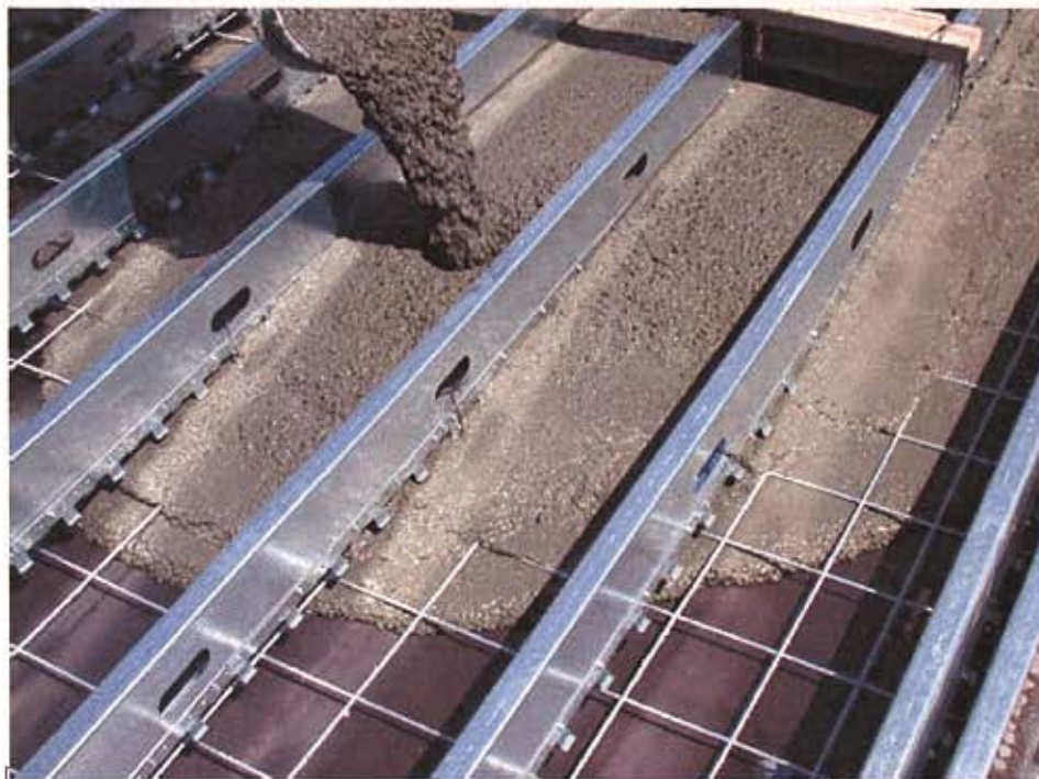
To make the thin-shell concrete panels, Y-shaped shear transfer strips are used to create composite action between the cold-formed steel studs and the concrete faces. Welded-wire mesh is used to reinforce the concrete.
