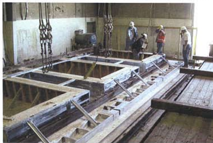
While the precast concrete is very thin, entrances and windows were recessed 30 inches to make the wall look thick and massive and create dramatic shadows.
