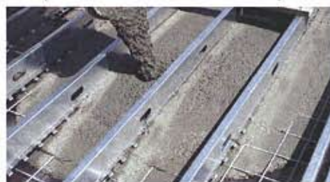
The light weight of the thin precast panels made it practical to transport and erect panels (above) up to 16 feet tall by 40 feet long. The concrete was poured (below) in a downward position and then rotated into a vertical position.
