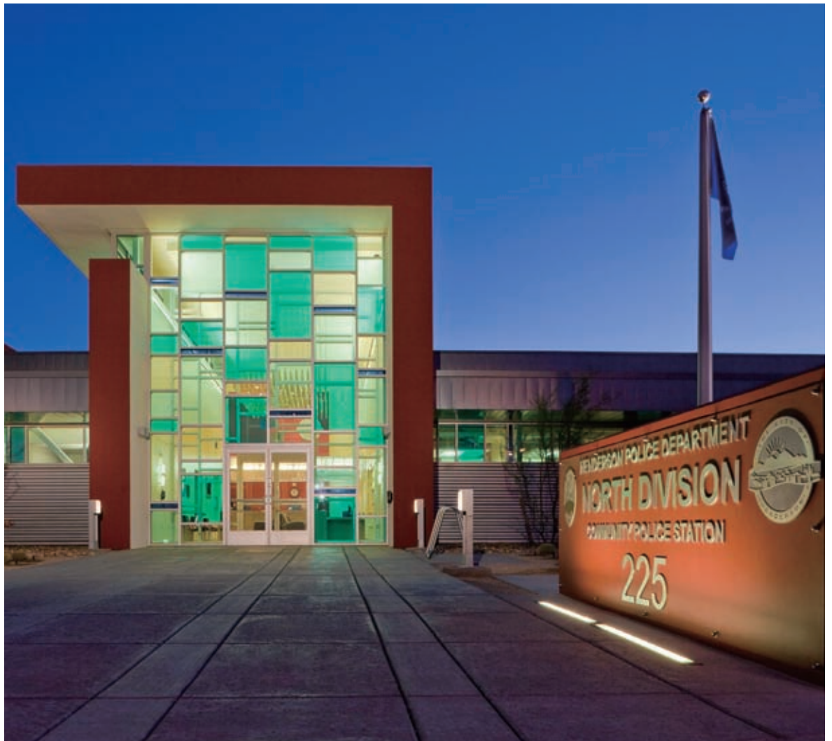
TOP, LEFT: TSKC Architects received its first contract with the Long Beach Port, for the Pier A project, in 1999. TOP, RIGHT: The Springs Preserve project in Las Vegas, is divided into two functional areas: a ticketing building with offices, a retail shop and cafe, and a gallery building with exhibits and a theater. RIGHT: TSKC served as the architect and interior designer for the Henderson Community Police Station.
