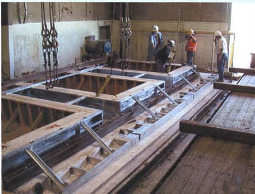
Panels used the Metal Stud Crete shear transfer strip to create a composite with a 2 1/2 in thick concrete face joined to cold-formed metal stud framing.
