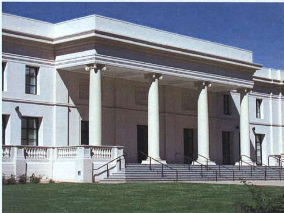
The Munger Research Center offers a contemporary reinterpretation of the neoclassical architectural detailing used throughout the Huntington Library and Gardens. Thin-shell precast concrete panels were used for exterior walls.
