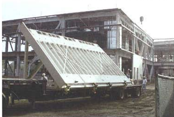
The large panels had to be shipped on a slanted easel at a 35-degree angle to be able to pass under a highway overpass. All panels traveled 80 miles without a crack.
