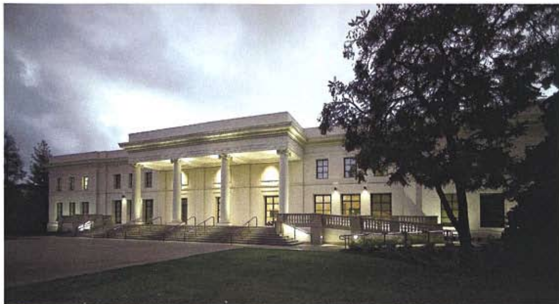
Exterior precast walls, which were installed in less than two months, accounted for just $1.5 million of the project's $20 million construction cost.
