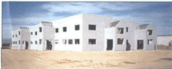
Above and right illustrate the erection process of the MetalStudCrete panels. Below is a view of the completed project which utilized approximately 10,000 sq. ft. of MetalStudCrete panels. Each one was 15' x 24'.
