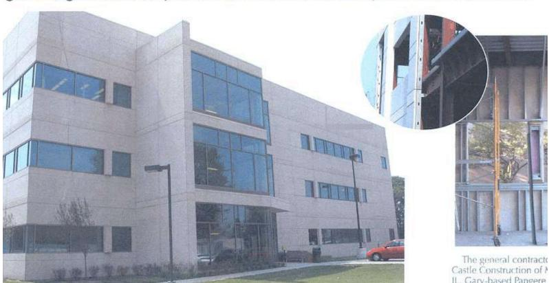
Sary, IN-On this particular ject at the Indiana University npus, two medical facilities utied Metal Stud Crete (MSC) panfrom Earl Composite Systems of indale, CA, as the exterior :losure system. The MSC panels.
