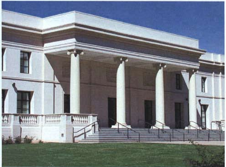
The Munger Research Center offers a contemporary reinterpretation of the neoclassical architectural detailing used throughout the Huntington Library and Gardens. Thin-shell precast concrete panels were used for exterior walls.
