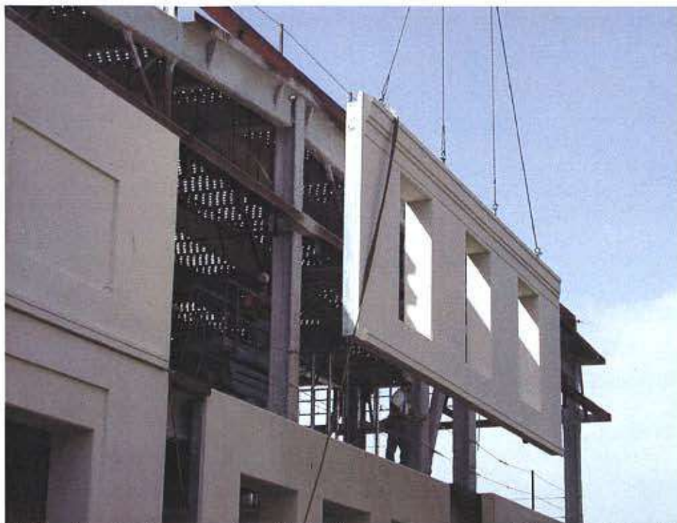
The light weight of the thin precast panels made it practical to transport and erect panels (above) up to 16 feet tall by 40 feet long. The concrete was poured (below) in a downward position and then rotated into a vertical position.
