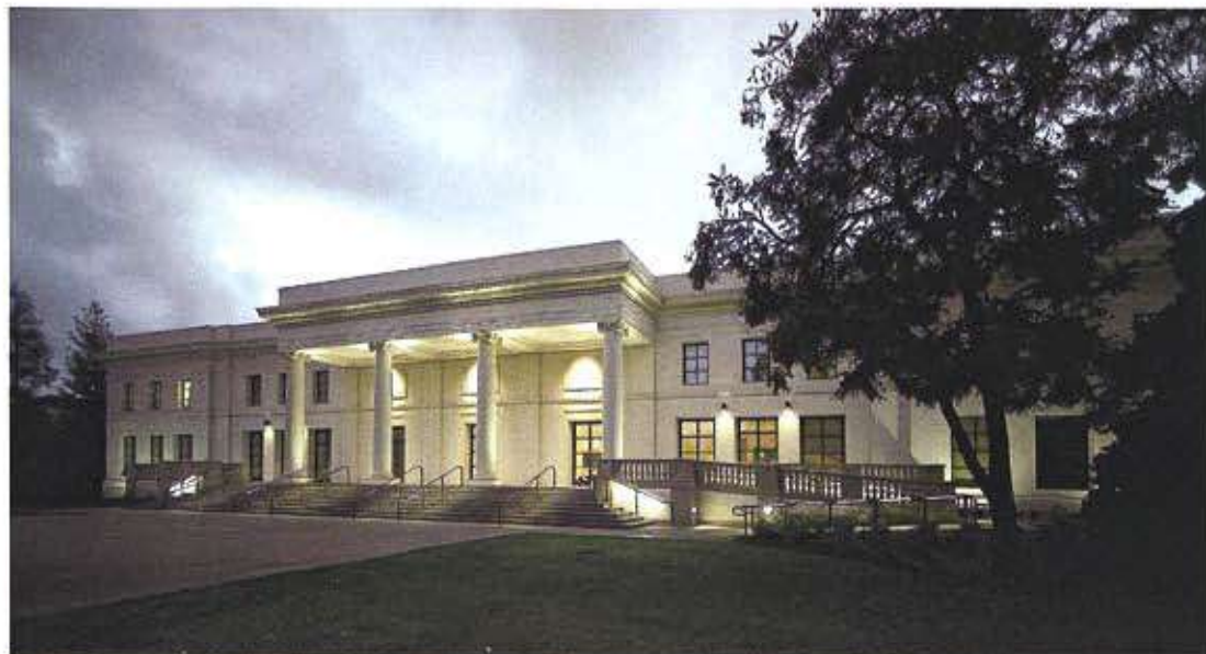
Exterior precast walls, which were installed in less than two months, accounted for just $1.5 million of the project's $20 million construction cost.
