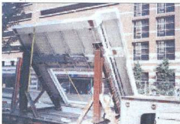
The backside of the precast Metal Stud Crete panels show the cold-formed steel stud framing used to support the 2 1/2-inch-thick precast concrete face. Metal framing provides space for utilities and insulation.
