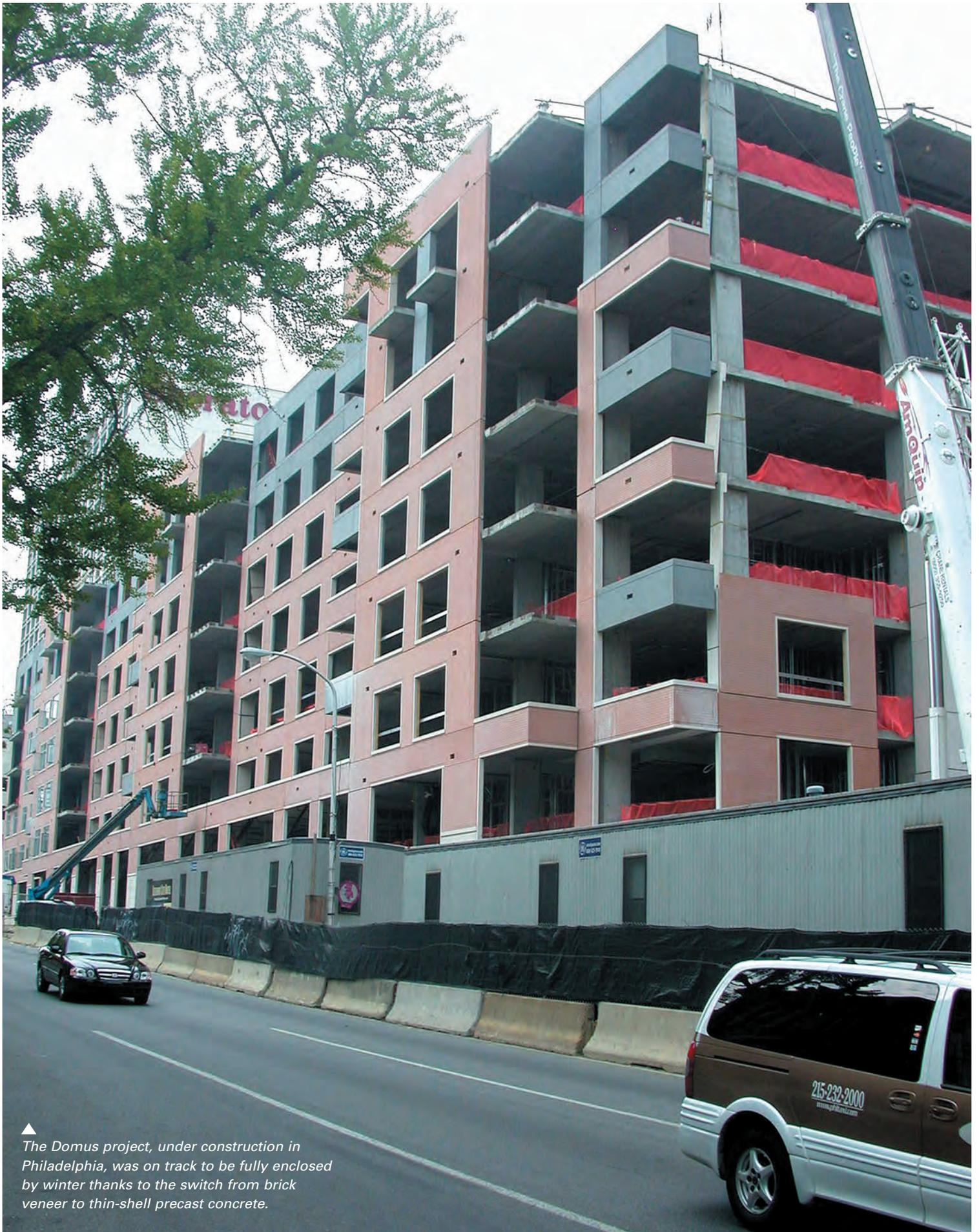
▲ The Domus project, under construction in Philadelphia, was on track to be fully enclosed by winter thanks to the switch from brick veneer to thin-shell precast concrete.
