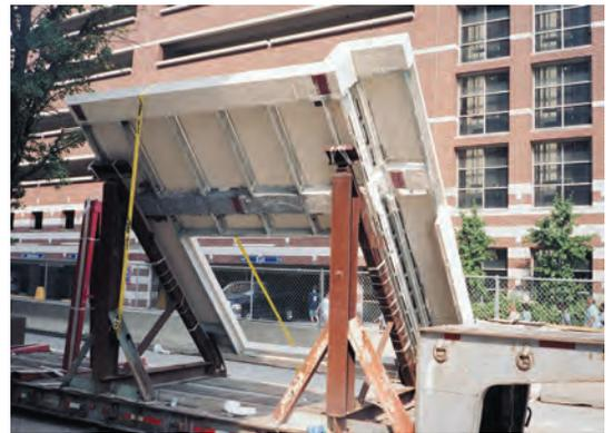
Clockwise from top right: The backside of the precast Metal Stud Crete panels shows the cold-formed steel stud framing used to support the 2 1/2-inch-thick precast concrete face. Metal framing provides space for utilities and insulation; the thin dark-red streak on the face of the panels is the integrally colored precast concrete only 2 1/2-inches thick. Additional beams were cast into the panels to provide connection points and a fire stop at the floor-to-wall connection.
