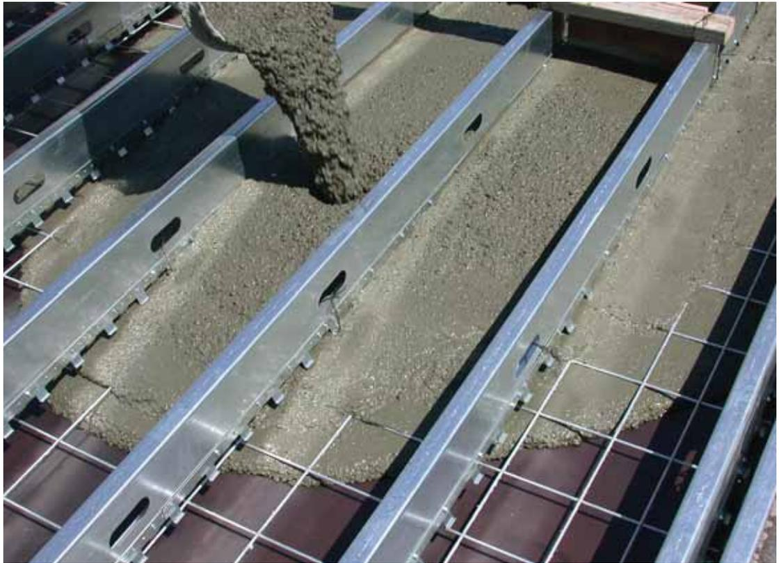
is that the system can be used by any precaster, and it saves time. Because of the reduced weight, overnight curing typically achieves sufficient strength for the assembly to be lifted out of the forms the next day, speeding the casting beds' cycle time as compared with conventional precast. Panels can then be moved to a storage position to continue curing before shipment.
